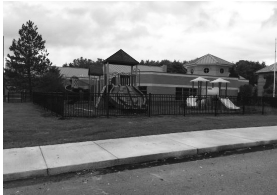
New Fence at Kindergarten Playground
