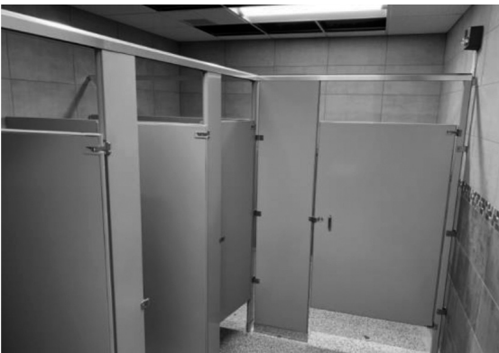
New Women's Restroom Renovation
