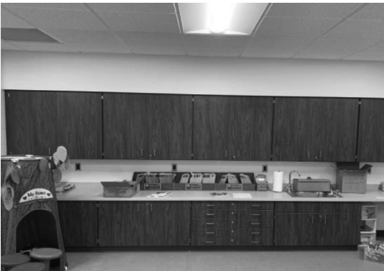
New Casework in Classroom Addition
