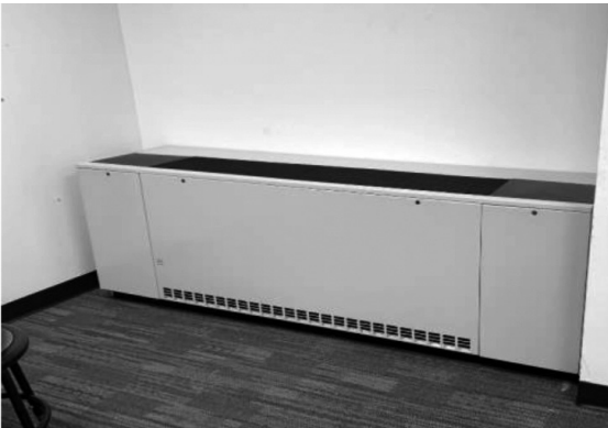
Unit Ventilator with Air Conditioning at Hiawatha
