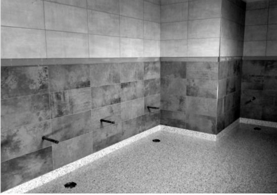
Toilet Room Wall Tile and Lighting at Central
