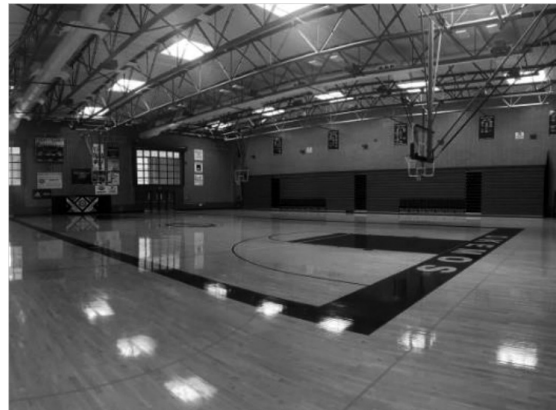
LED Lighting at High School Gymnasium
