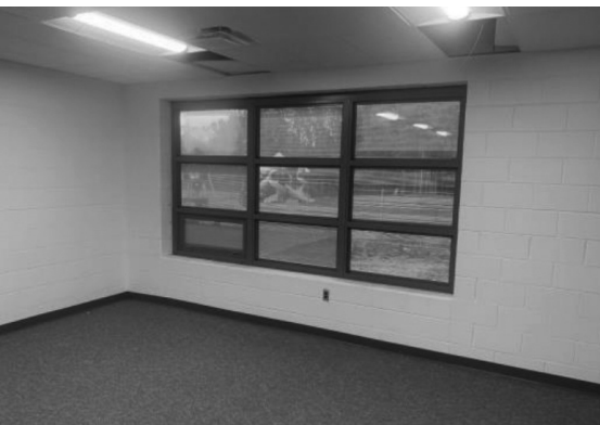
West Addition Exterior Window
